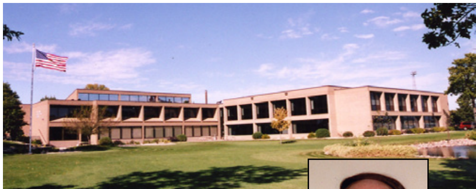
North Star Mutual Headquarters Cottonwood, MN
